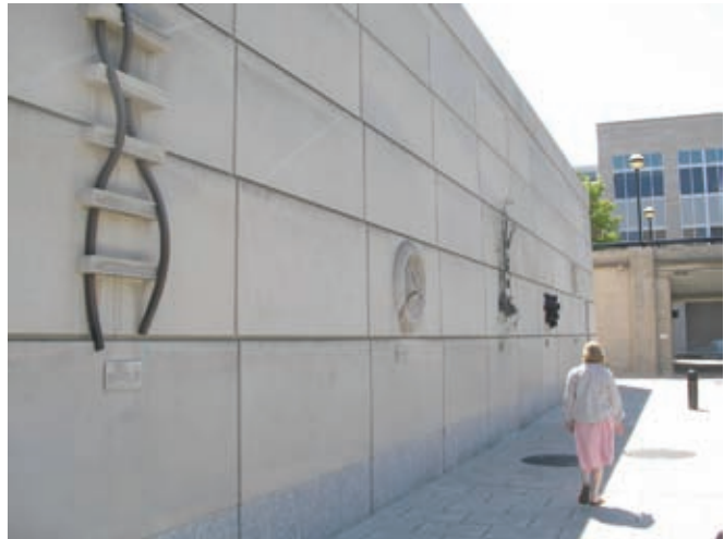
US 1.5.1: Walls and facades of the Indiana State Museum incorporate artwork from every Indiana county and help transform an otherwise monolithic wall into a site amenity.
