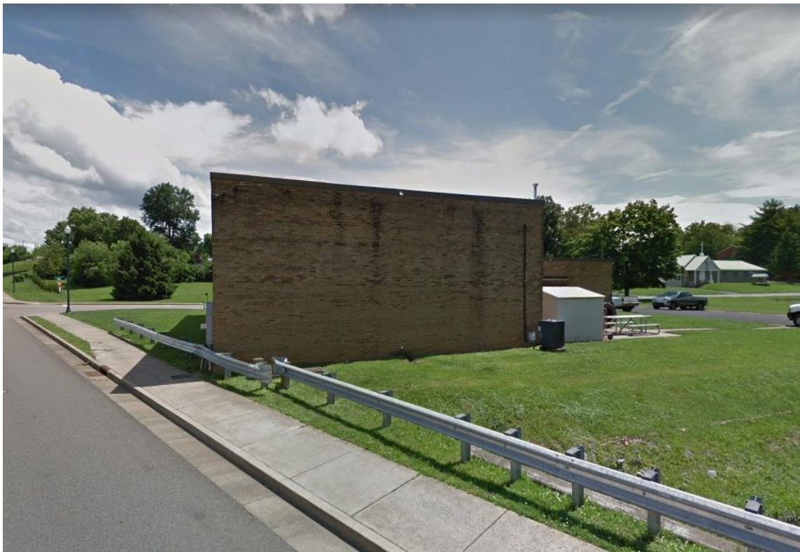
Back Wall - Market Street Side
