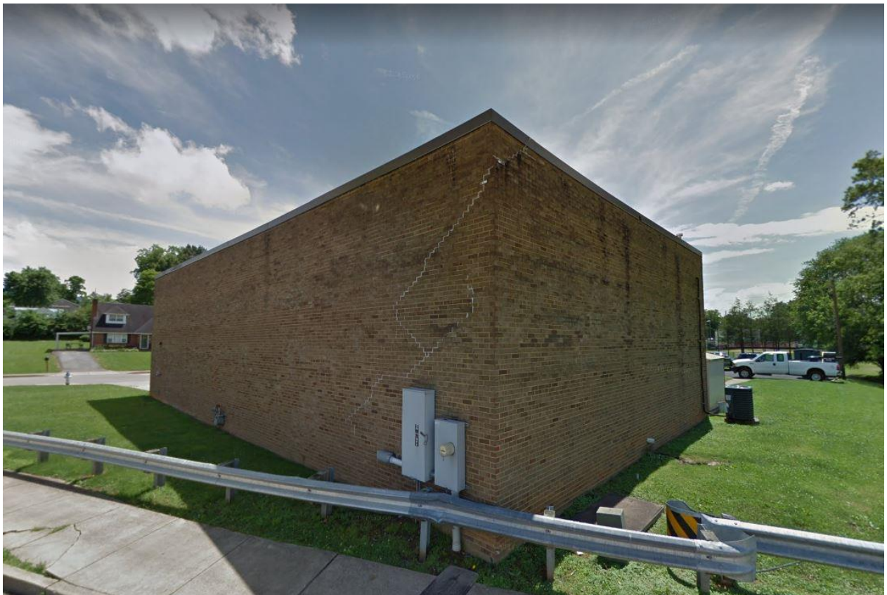
Side & Back Walls
