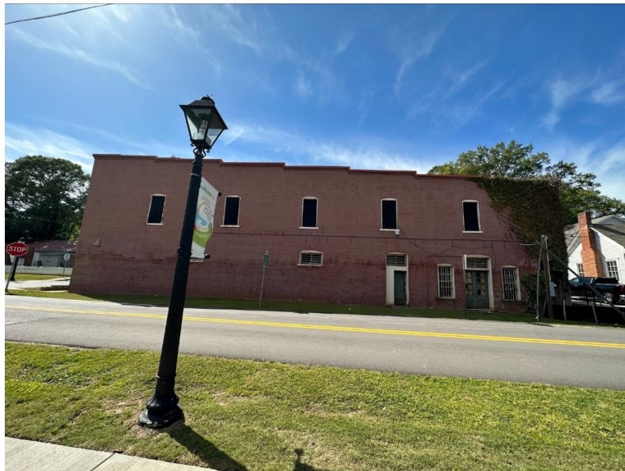
Photo of mural wall, in its current condition, prior to renovation.
