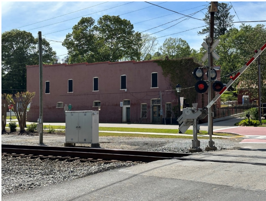
Photo of mural wall, in its current condition, prior to renovation. The Norfolk Southern railroad crossing in shown in the foreground.
