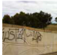
Decorative Sound Walls
