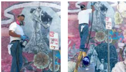
MURALSHIELD being applied with HVLP sprayer
