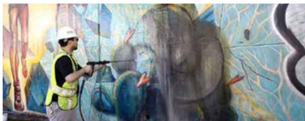
Cleaning graffiti after using MURALSHIELD in conjunction with WORLD'S BEST COATING.
